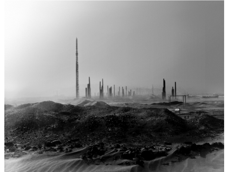
Figure 3-9 Construction of POSCO at Yeongilman Bay Wasteland Source: The Asia Business Daily , October 22, 2012.
