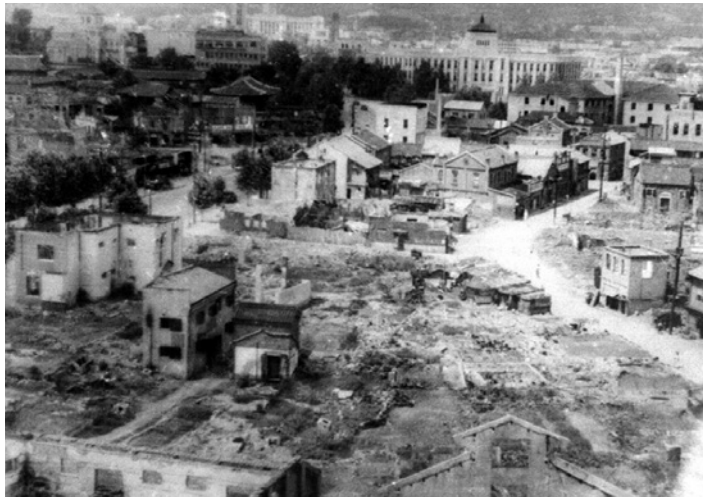
Figure 1-1 Buildings in Seoul destroyed by bombing Source: National Archives of Korea.
