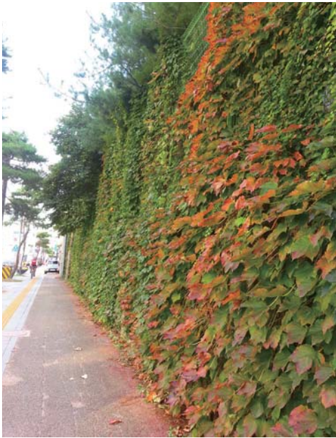
Photo 15 Forestation of Roadside Cutting Area
